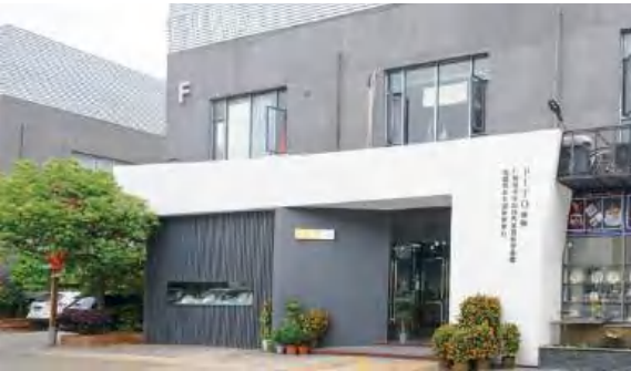
GBI / Catering Products Experience Center / Consulate kitchen
