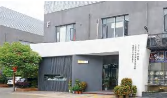
GBI / Catering Products Experience Center / Consulate kitchen
