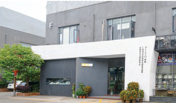
GBI / Catering Products Experience Center / Consulate kitchen
