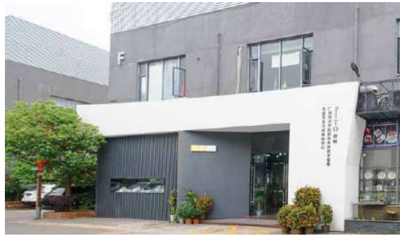
GBI / Catering Products Experience Center / Consulate kitchen
