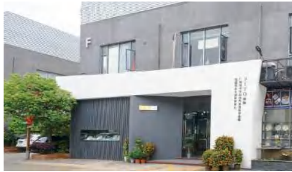
GBI / Catering Products Experience Center / Consulate kitchen
